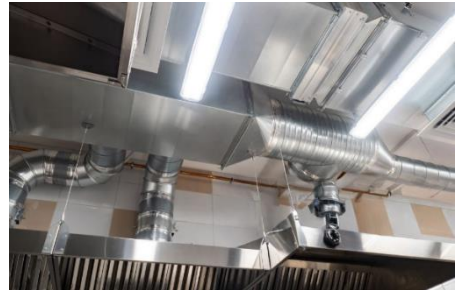
4-4 Kitchens Shall Be Equipped with an Air Make-up System
